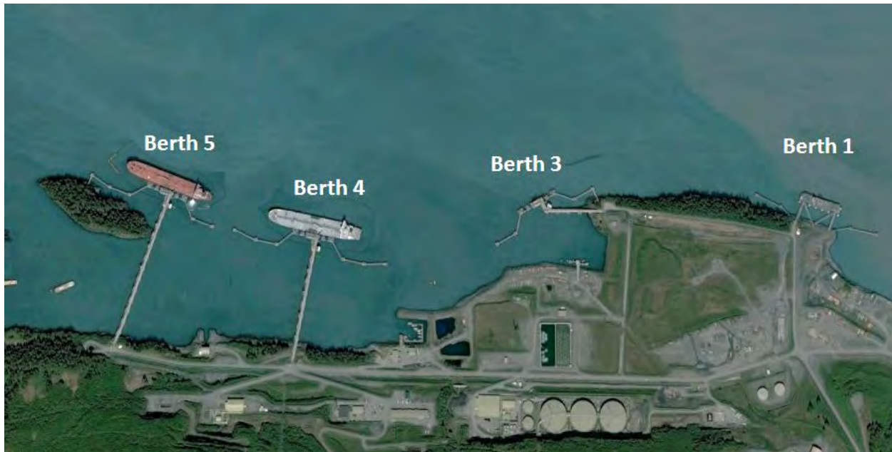
Figure 3. Aerial view of berths at Valdez Marine Terminal (Google Earth)
