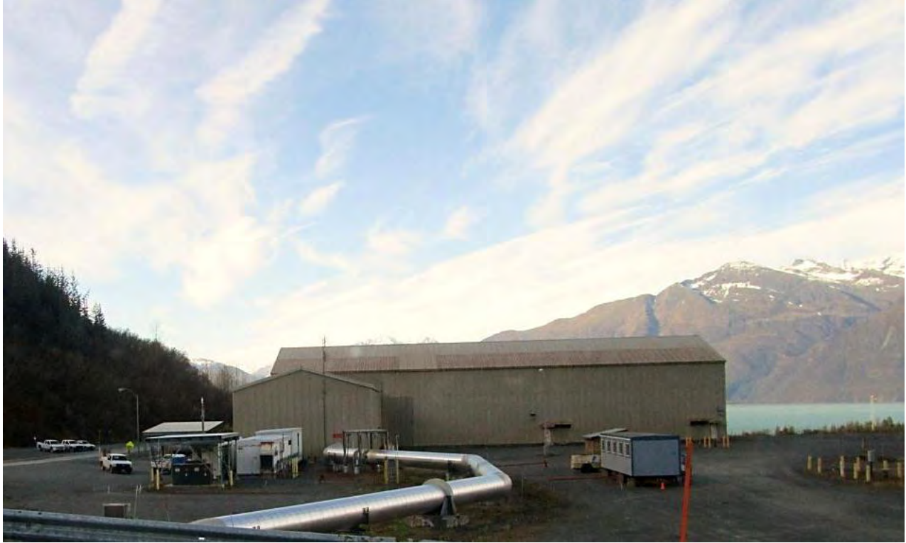
Figure 2. The southern end of the 800 mile-long Trans Alaska Pipeline at Valdez Marine Terminal (photo by M. Kartezhnikova).
