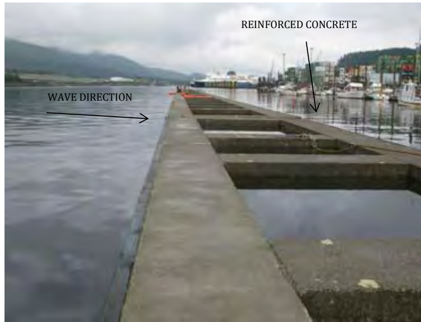
Figure 19. Alaskan floating breakwater design at Bar Point Harbor in Ketchikan, Alaska (photos by Lt. Jon-Paul Navarro, Arctic Engineer, 2010)
